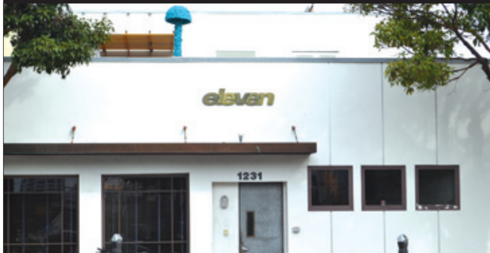
Stu Mitchell was the first person to identify the photo as part of the building located at 1231 Lincoln Blvd. He wins a prize from the Daily Press.
